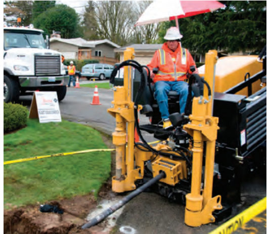
Natural gas main upgrade work in Bellevue
